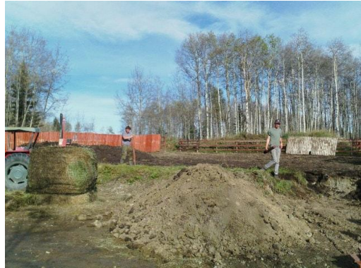
Removing existing corral fencing.
