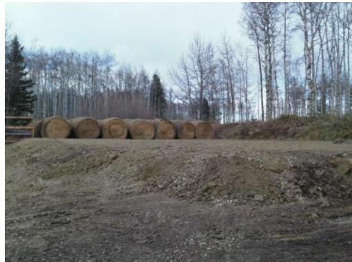
Clay and gravel moved to level off the site.
